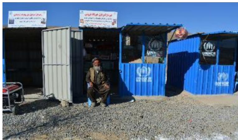
Picture of the metallic shops for 10 vulnerable Returnees and IDPs in Narkh LAS – Maidan Shahr-Wardak
